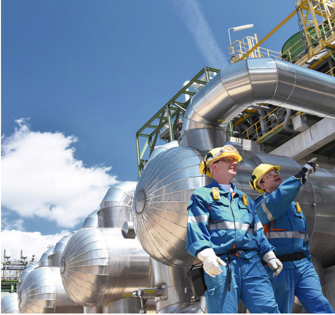
Refinery acceptance of crude oil is normally less than 1% Basic Sediments & Water (BS&W)
